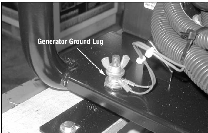
Figure 13 - Grounding the Generator
